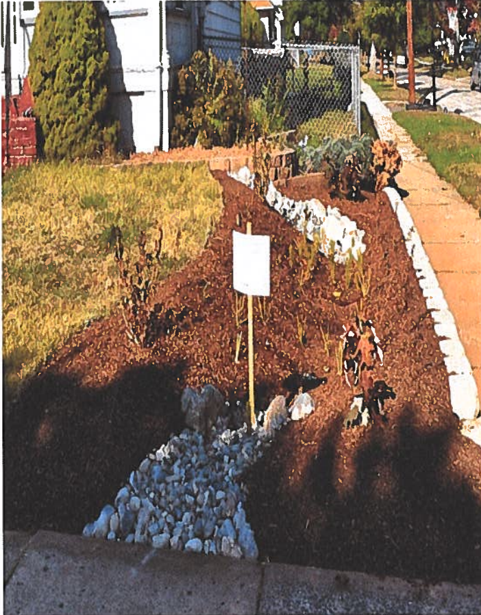
Laying down stone helps prevent erosion and contain sediment.
