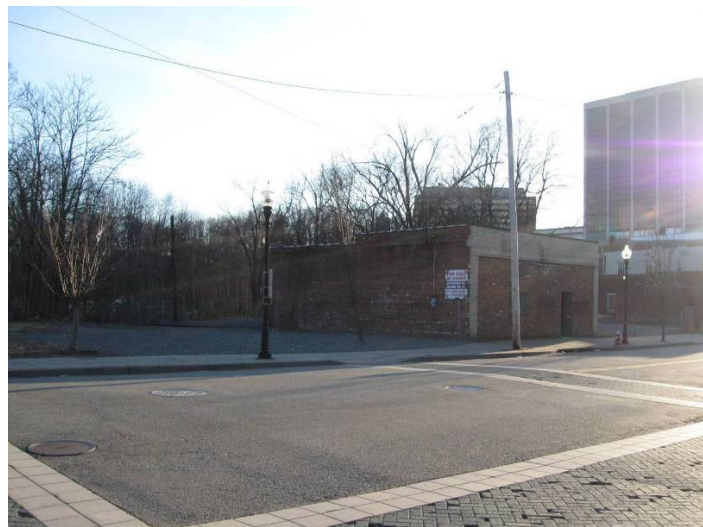
Figure 26: Area of Concern #6 Building
