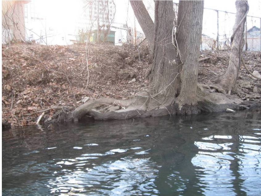
Figure 10: Area of Concern 2 Tree 4 to Remain
