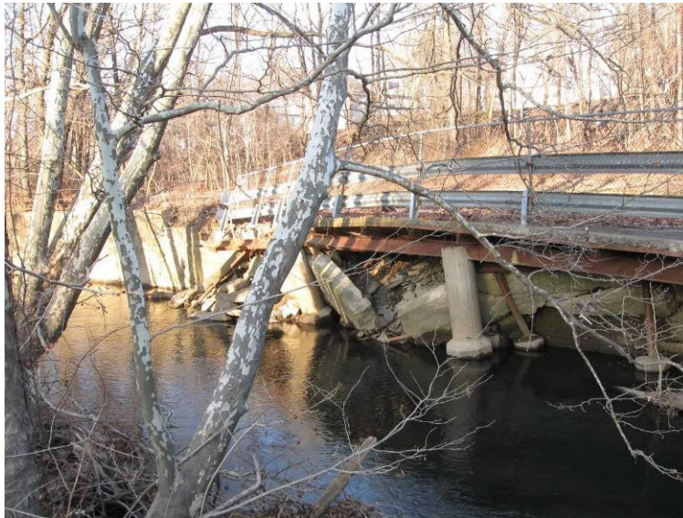
Figure 31: Area of Concern #7 Collapse of the Platform
