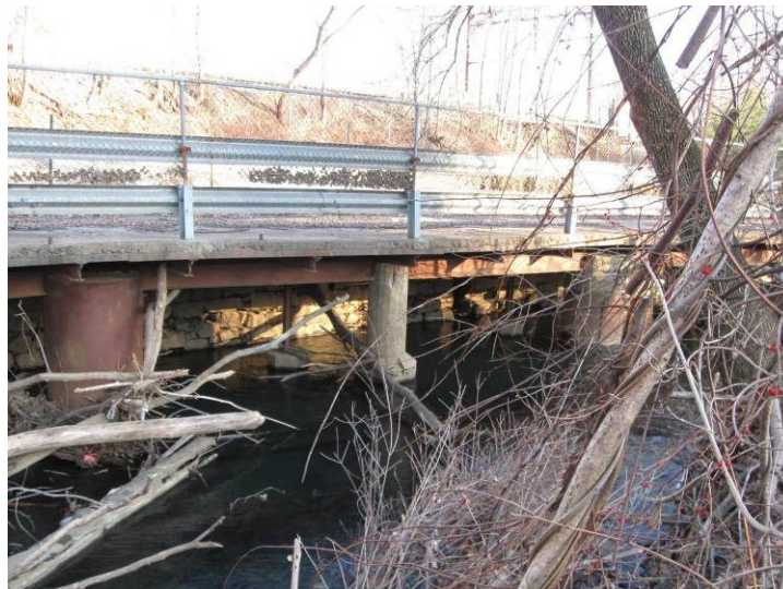
Figure 29: Area of Concern #7 View of the Platform and Columns
