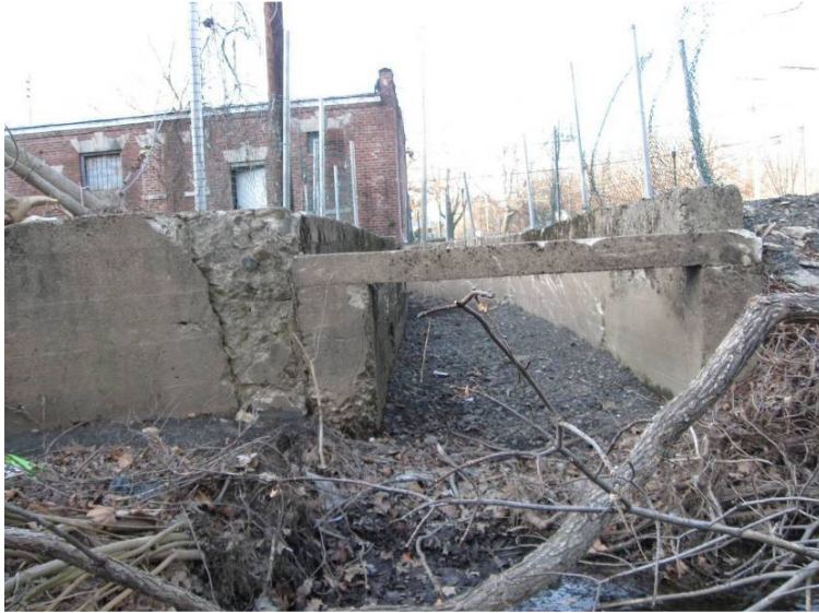
Figure 27: Area of Concern #6 Concrete Channel
