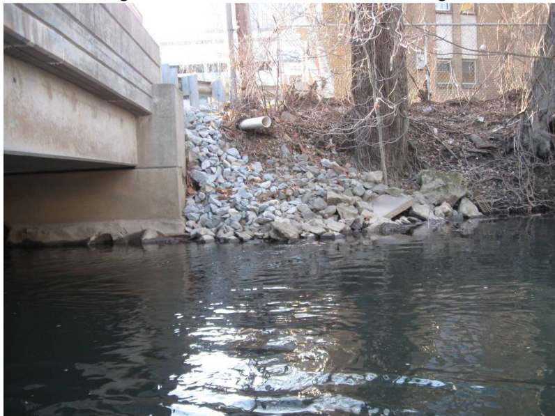
Figure 5: AOC #1 near Center Street Bridge
