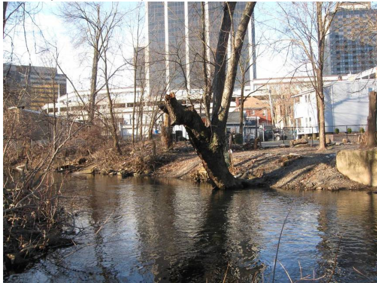
Figure 8: Area of Concern #2 Upstream end near the Concrete Retaining Wall.
